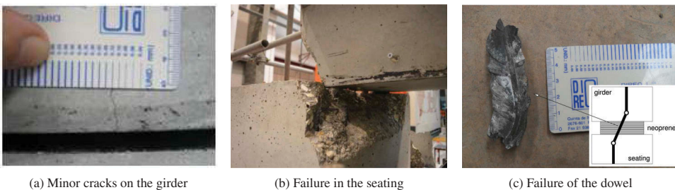
Figure 8. Damage observed after the experimental cyclic test.
