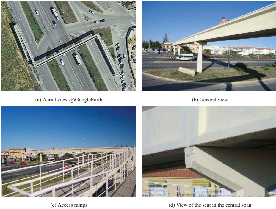
Figure 2. Pedestrian crossing PP2787 across the IC4 Portuguese highway.
