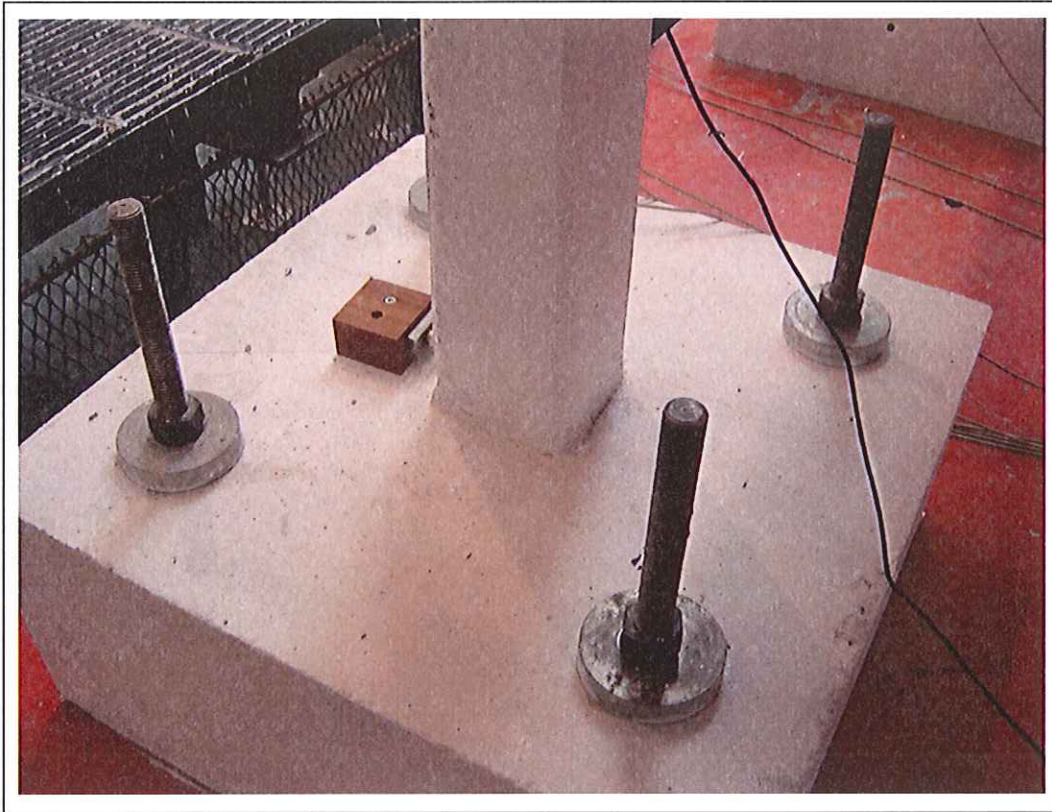
Figure F-33: Detail of the base of the column C3 after the test
