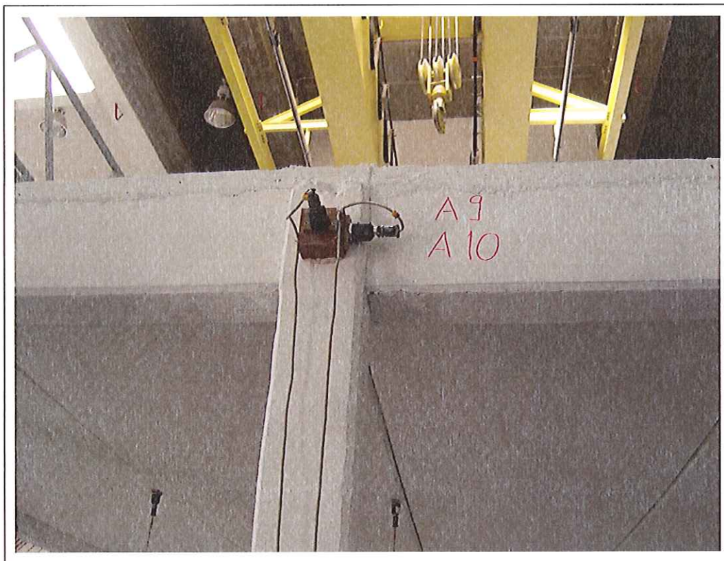
Figure F-18: Detail of the beam-column connection after stage 02 (J11-Long.)
