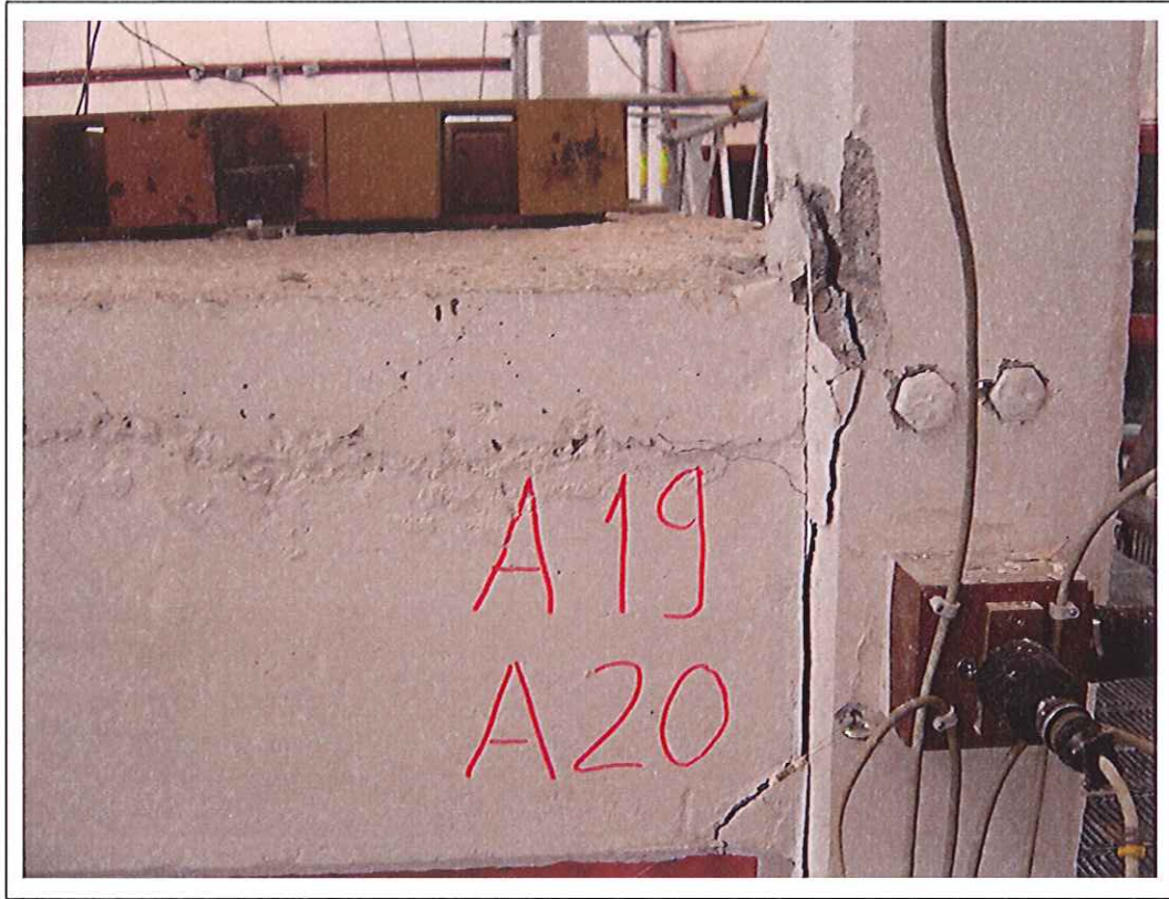
Figure F-27: Detail of the beam-column connection after the test (J6-Long.)
