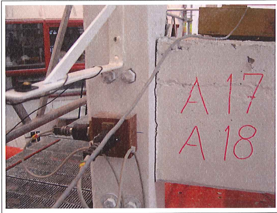
Figure F-29: Detail of the beam-column connection after the test (J1-Long.)
