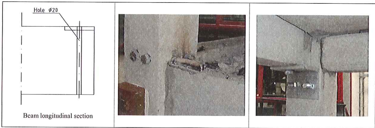
Figure 3-4: Beam-column connection type #2.
