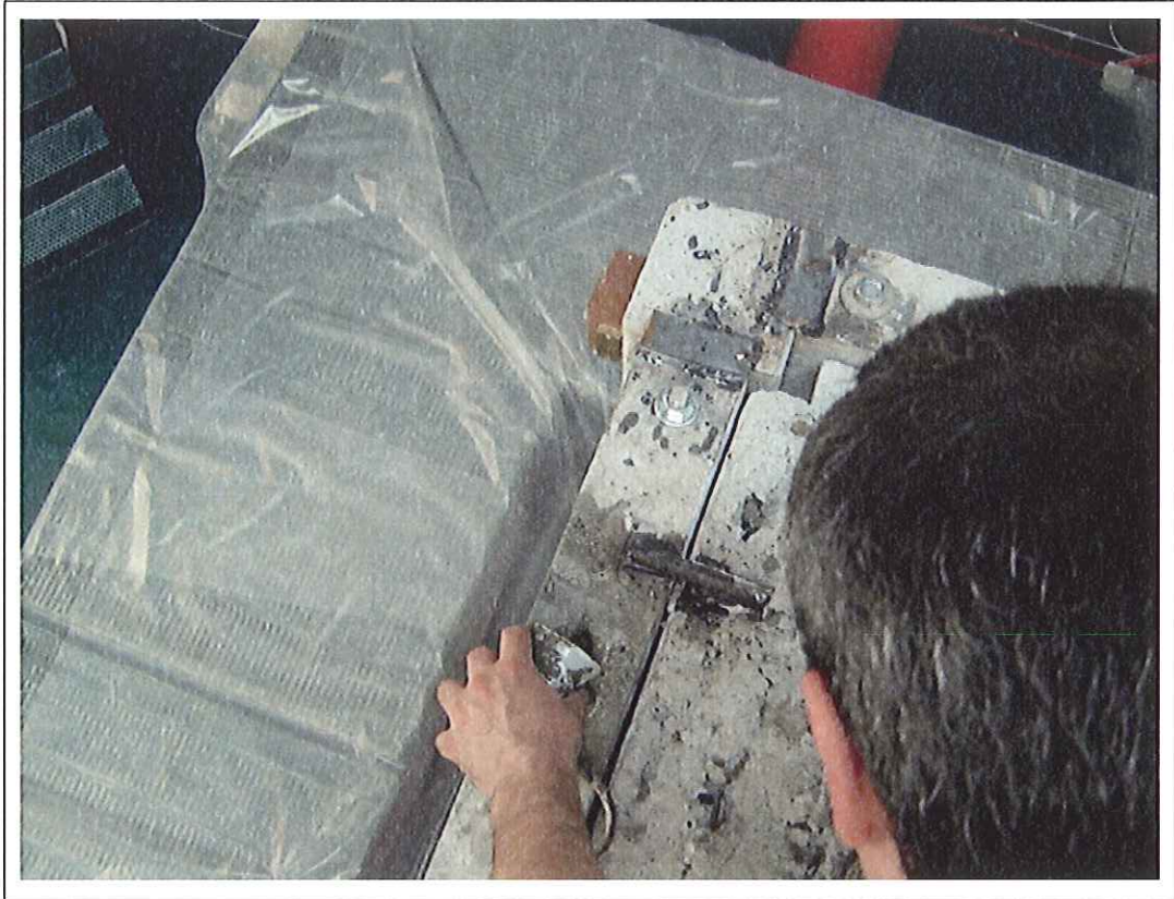
Figure F-7: Detail of the joint sealing operation (J7-Long.)
