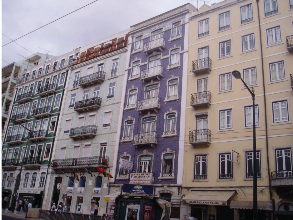
Figure 3.5 – Masonry old buildings, “Gaioleiros” [after Sousa, 2005].
