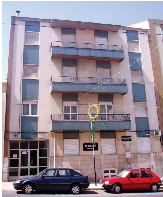
Figure 3.8 – RC buildings after RSCCS code and before RSA [after Sousa, 2005].
