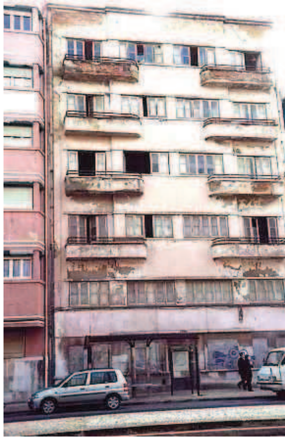
Figure 3.6 – Masonry buildings with unreinforced brick with RC floors, “placa” in bad state of preservation.
