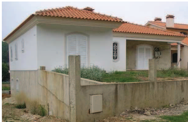
Figure 3.7 – Confined masonry building [after Sousa, 2005].
