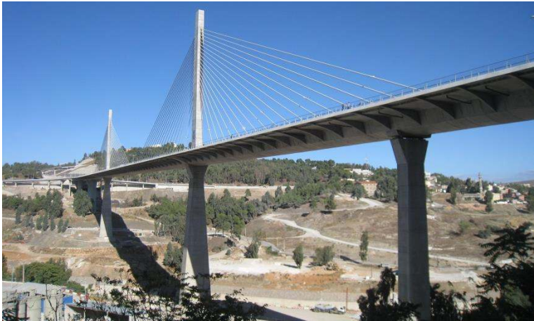
Figure 3: General view of Salah Bey Viaduct
