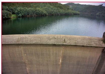
Figure 25: Inclined photograph of the spillway on the crest of Bouça dam
