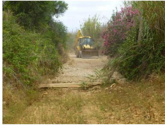
Figure 9 – Levelling of Rio Seco bed
