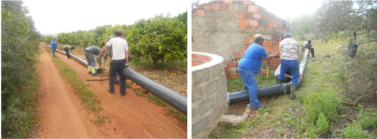
**Figure 92 – Illustration of the work to install the 1.4 km pipeline from SJS2 well to CB well**
