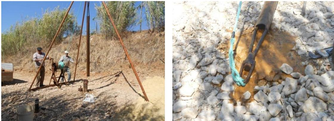
Figure 12 – Piezometer and well development
