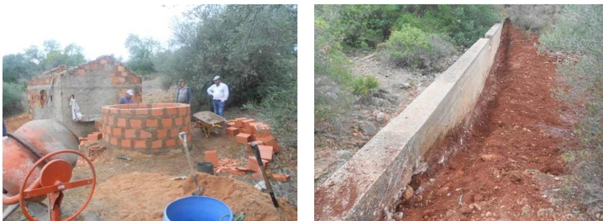
**Figure 76 – Cerro do Bardo large well and weir (Aivados dam) rehabilitation**
