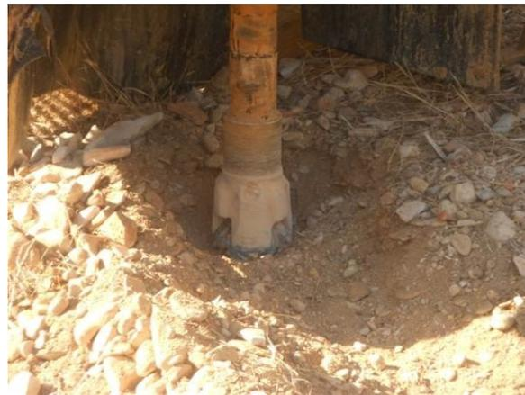
**Figure 14 – Rotation with direct circulation**
