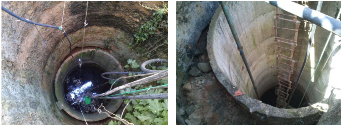
Figure 17 – Traditional large diameter wells potentially suited for injection of harvested water
