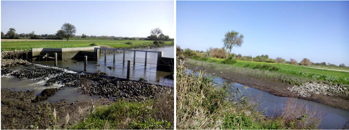
Figure 2.7 – Site 3: Weir of the Risco river (November 26, 2015)
