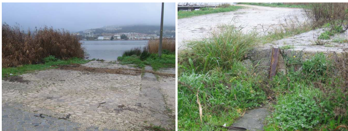
Figure 2.12 – Site 11: Old dock of Vila Franca de Xira (January 21, 2016)
