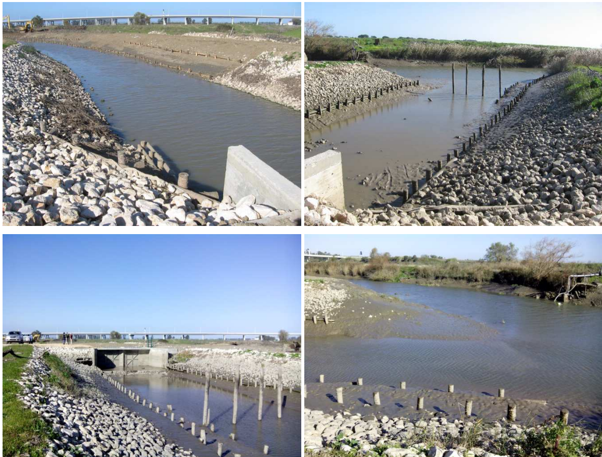
Figure 2.8 – Site 4: Confluence of the Risco and Sorraia rivers (November 26, 2015)
