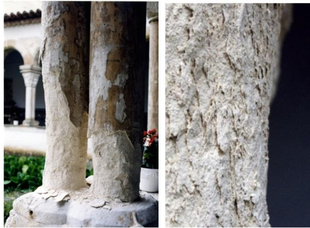
Fig. 3 – Ançã stone columns at the cloister of Santa Cruz Monastery (left) and detail of their decay pattern (courtesy of J. Delgado Rodrigues).
