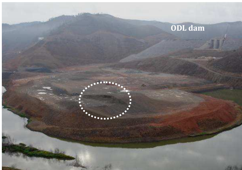
Figure 5.1 – Location of the borrow area used for the construction of Odelouca (ODL) dam, where materials have been collected.
