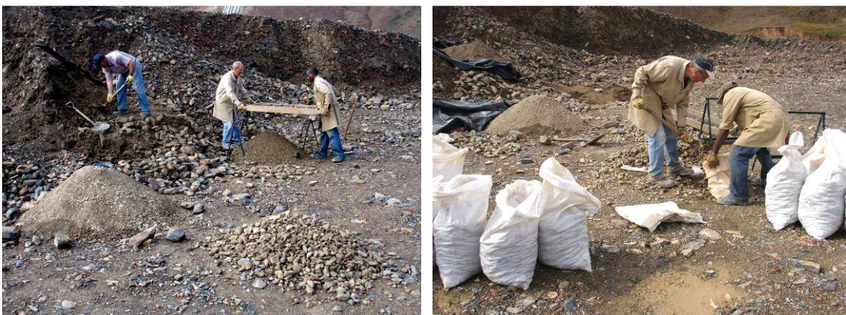
Figure 5.2 – Sieving and bagging of materials in the ODL dam borrow area.
