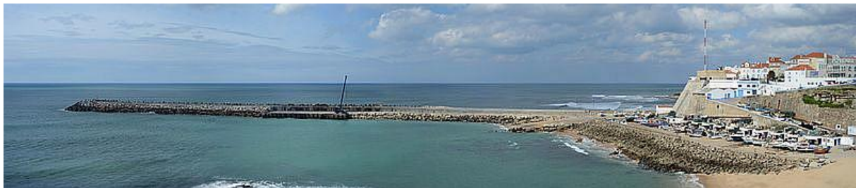
Figure 2 – Breakwater of the port of Ericeira after the rehabilitation.
