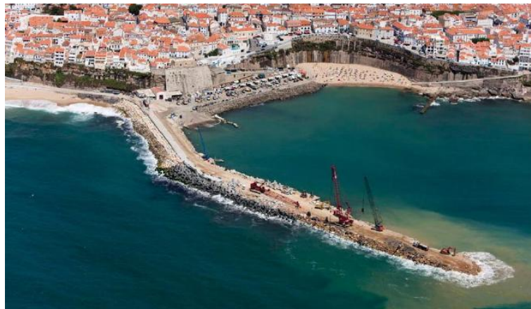
Figure 1 – Reconstruction of the breakwater of the port of Ericeira.
