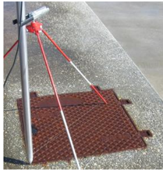
Figure 9 – Southwest corner of a manhole being coordinated.
