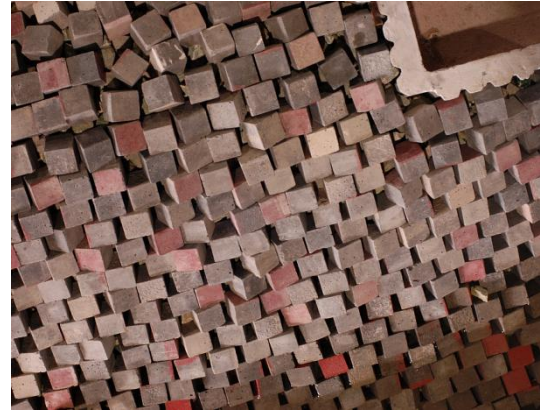
Figure 17 – Blocks of concrete.
