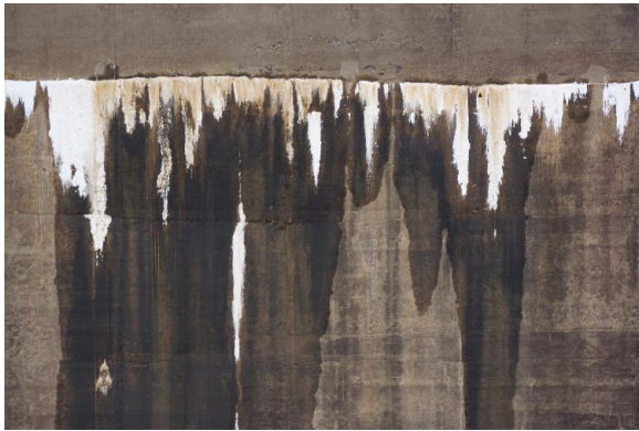
Figure 7: Flight A. Crack n.º2 photographed with a focal length of 50 mm.
