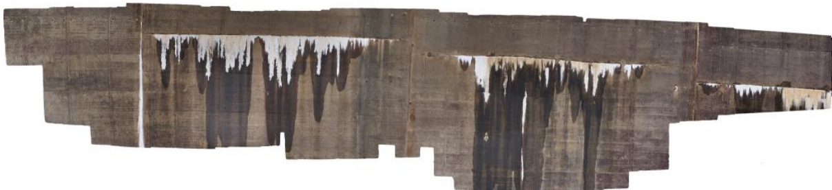
Figure 9: Image generated by Skyeye using software VisualSFM and photos of flight A.
