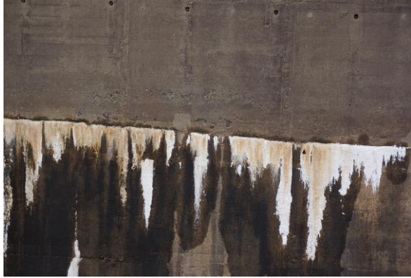
Figure 1: Horizontal photograph of the downstream wall of Bouçã dam.
