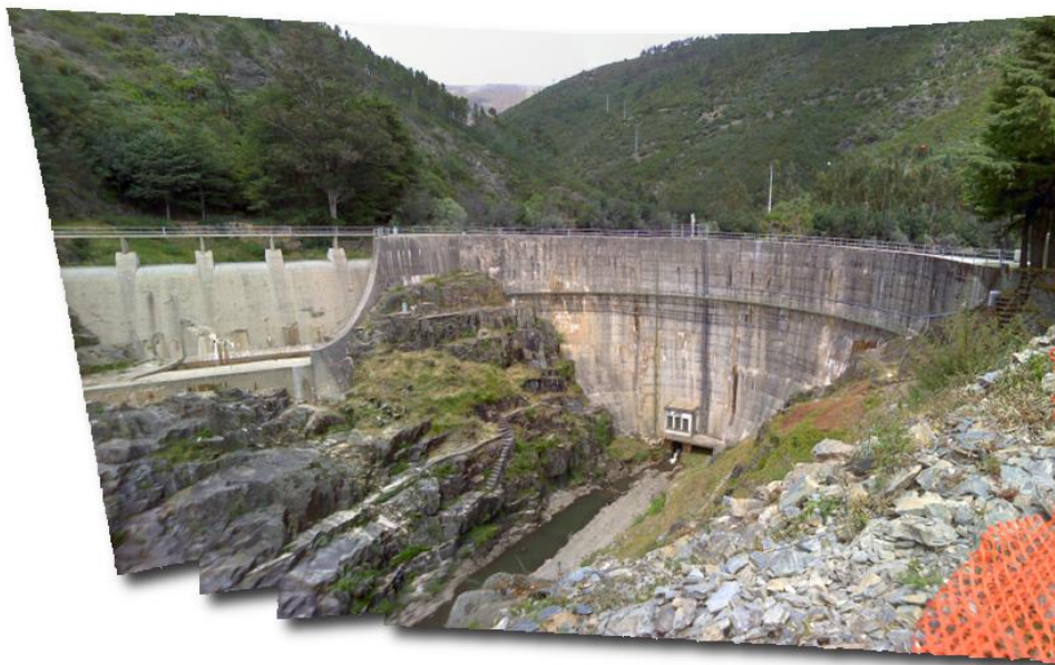
Figure 5: Panoramic image of Alto Ceira dam
