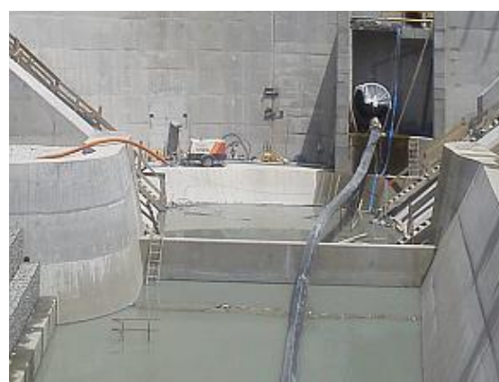
Figura 16: Visible image of the same area.
