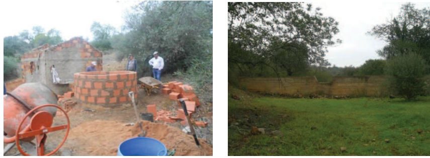
Fig. 6. Cerro do Bardo well and Aivados dam (PT2_6) (Leitão et al. , 2015)
