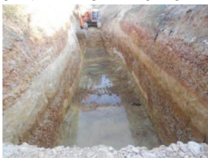
River basin excavation: August 2014
