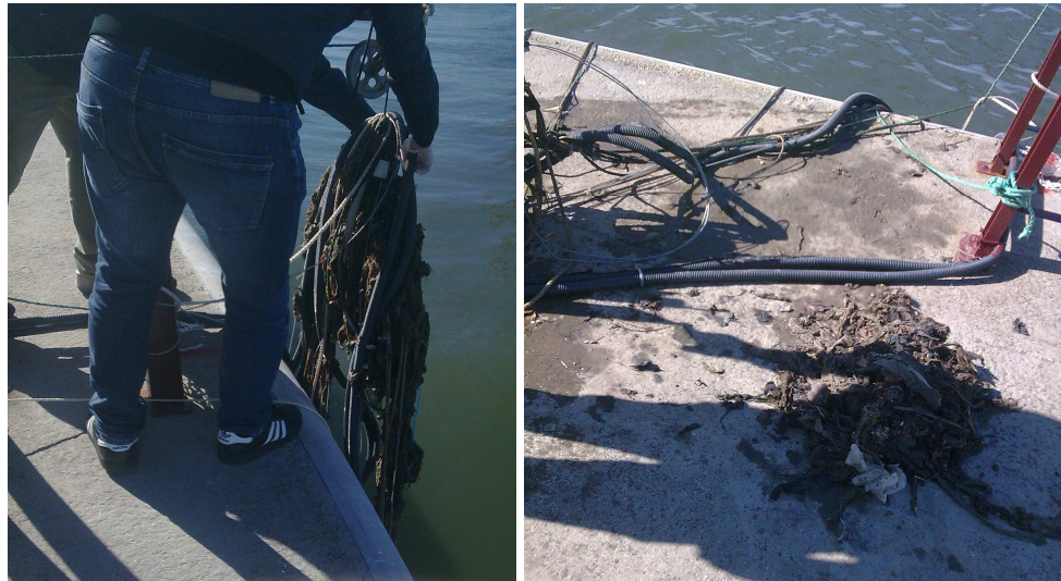
Figure 9 – Trash removed from the receiving waters on-line monitoring station during an out-of-schedule cleaning after an extreme rain event (November 30, 2013).
