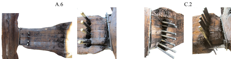
Figure 11. Connections A.6 and C.2 after the fire tests.
