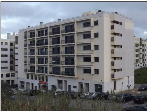
Figure 5. A building of the urbanization where the survey was applied
