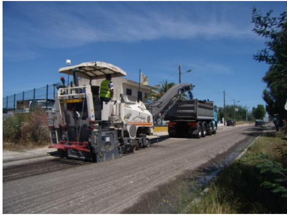
Fig. 1. Milling the old pavement
