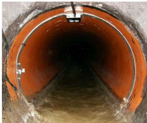
Figure 5.2: Flow measurement using the velocity-area method
