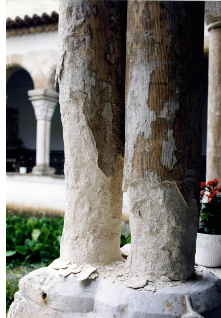
Santa Cruz Monastery (1132-1223), Coimbra – courtesy of J Delgado Rodrigues
