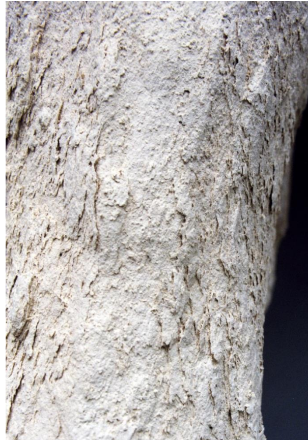
Columns at the cloister of Santa Cruz Monastery (1132-1223), Coimbra, Portugal, with delamination of Ançã limestone – courtesy of J Delgado Rodrigues
