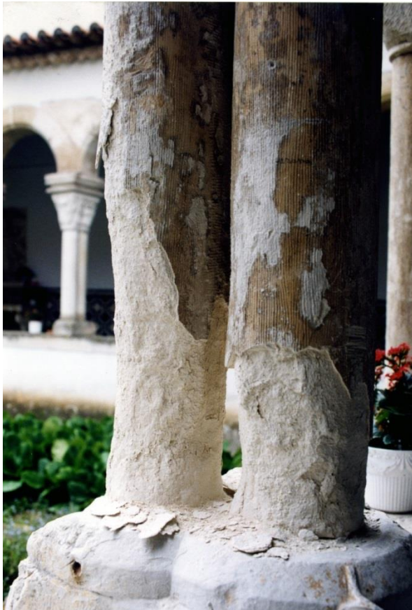
Columns at the cloister of Santa Cruz Monastery (1132-1223), Coimbra, Portugal, with delamination of Ançã limestone – courtesy of J Delgado Rodrigues
