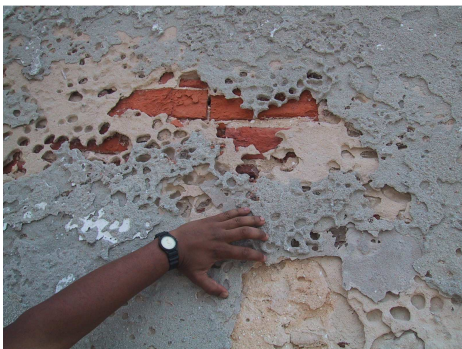
Fig.8 - Alveolization of render on the adjacent building N façade
