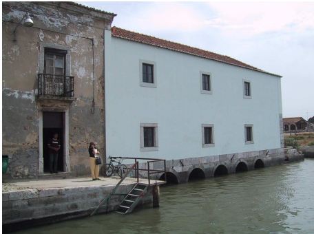
Fig.1 - Tide-mill (right) and adjacent building (left) – northern façades
