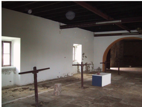
Fig. 3- Tide-mill: ground floor
