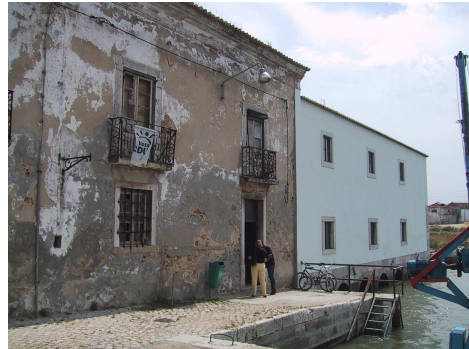
Fig. 1- Adjacent building (left) and tide-mill (right) – northern façades
