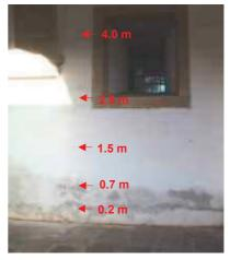
Fig. 16 – Moisture content profile of the NE wall
