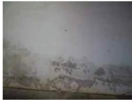
Fig.7 - Cloister gallery: damage of the render/paint system at the base of a wall (2003-11-27)
