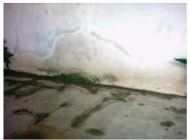
Fig. 9 – Moss and moisture spots on the base of a wall and on the pavement (2004-02-05)
