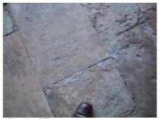
Fig. 12 – Efflorescences on stone pavement (2004-02-05)
