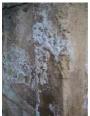
Fig. 10 – Efflorescences on stone (2004-01-08)
