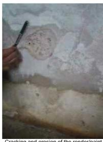
Fig. 8 – Cracking and erosion of the render/paint system (2004-01-08)
