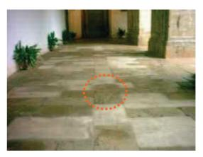
Fig. 15 – Liquid water on the vaults and pavement stones (2004-01-08)
