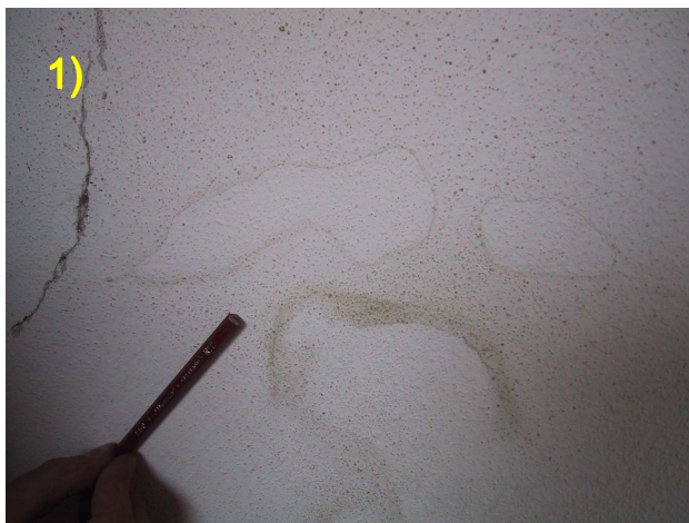
Fig. 16 – Often damage seems to start at cracks
