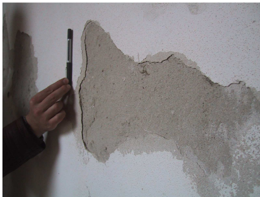
Fig. 9 – Detachment of the render superficial coat (2004-01-08)
