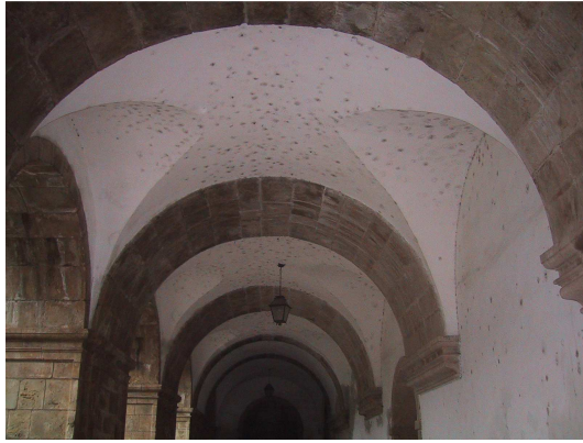
Fig. 11 – Unidentified biological development on the upper part of the walls and on the vaults render (2004-01-08)
