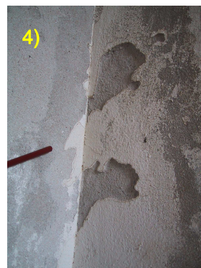
Fig. 17 – Evolution of damage starting from dry moisture spots. The dark lines may represent a microfissure
