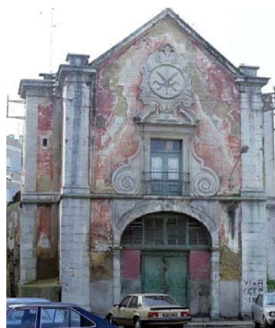
Fig. 6.21 – São Sebastião Church: NE (front) façade in 1999
