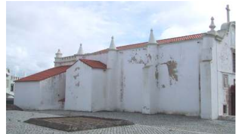
Fig. 6.4 - Salvas Chapel, NW façade October 2003
