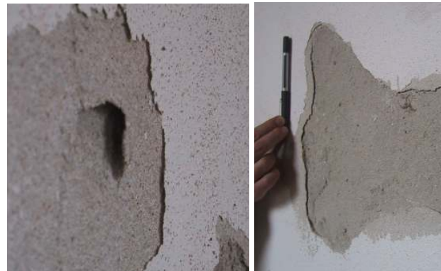
Fig. 6.18 – Sta. Clara: in some cases, damage starts by the bulging and further detachment of a thin surface layer of the render, accompanied by peeling of the paint, without the presence of efflorescence
