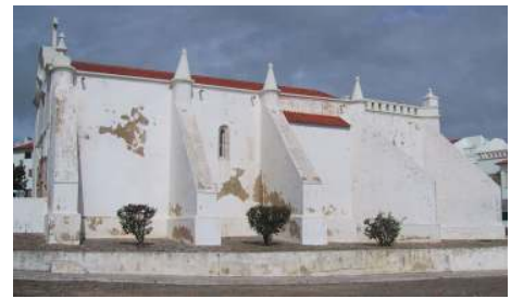
Fig. 6.3 –Salvas Chapel, SE façade, which faces Sines harbour, October 2003
