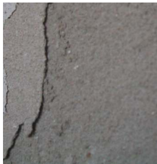
(g) Exfoliation (layering of material with non-laminated structure, in this case, the surface coat of the render) – Sta. Clara-a-Nova Monastery, Coimbra, 2005
