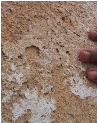
(e) Scaling of lime-wash / lime-render system – Torre das Cabaças, Santarém, 2002
