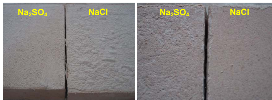
Fig. 5.37 - Damage on the unpainted stone specimens at the end of the first crystallization experiment: efflorescence (left), cleaned stone surface (right)
