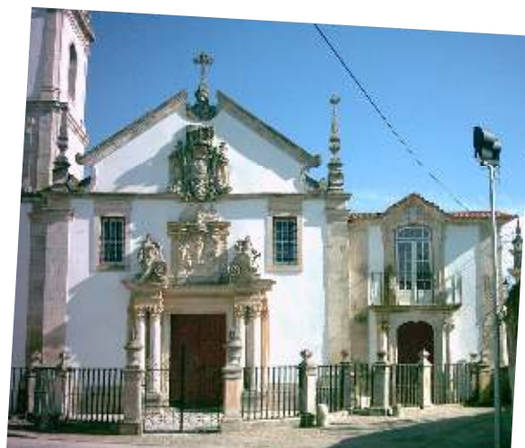
Fig. 6.11 - Pereira Misericórdia, West façade: tower (left), church (centre), Despacho House (right)
