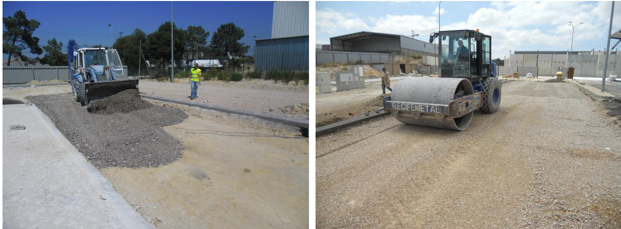
Figure 3: Construction of the experimental sections.
