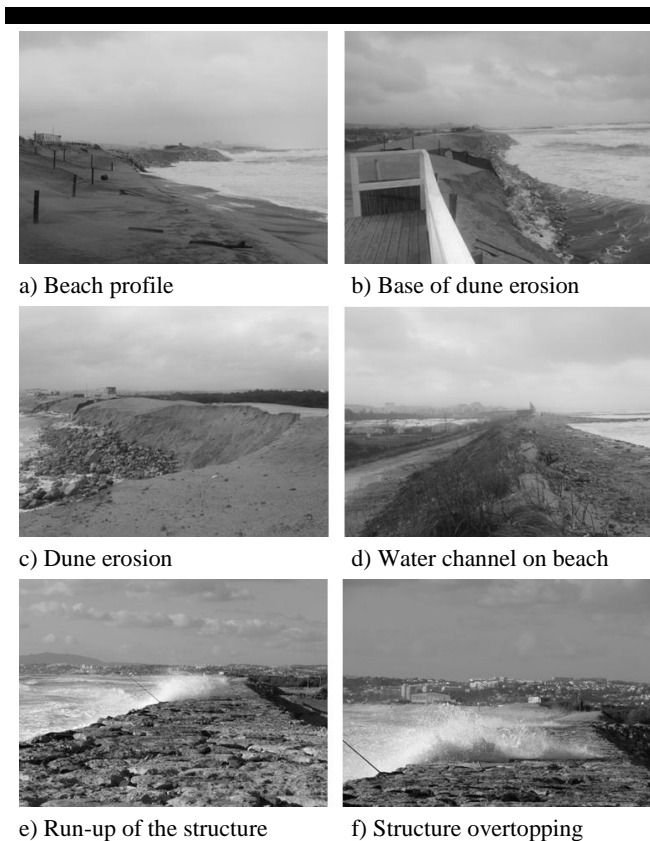
Figure 2. Effects of the 27.02.2010 storm at S. João da Caparica beach.
