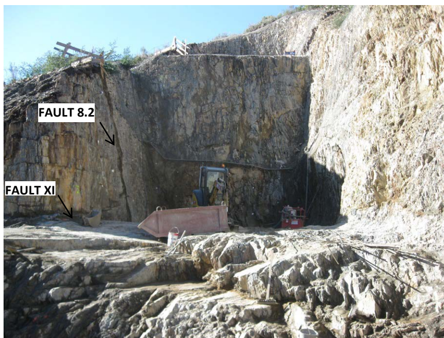
Figure 7 - Right abutment after complementary excavation
