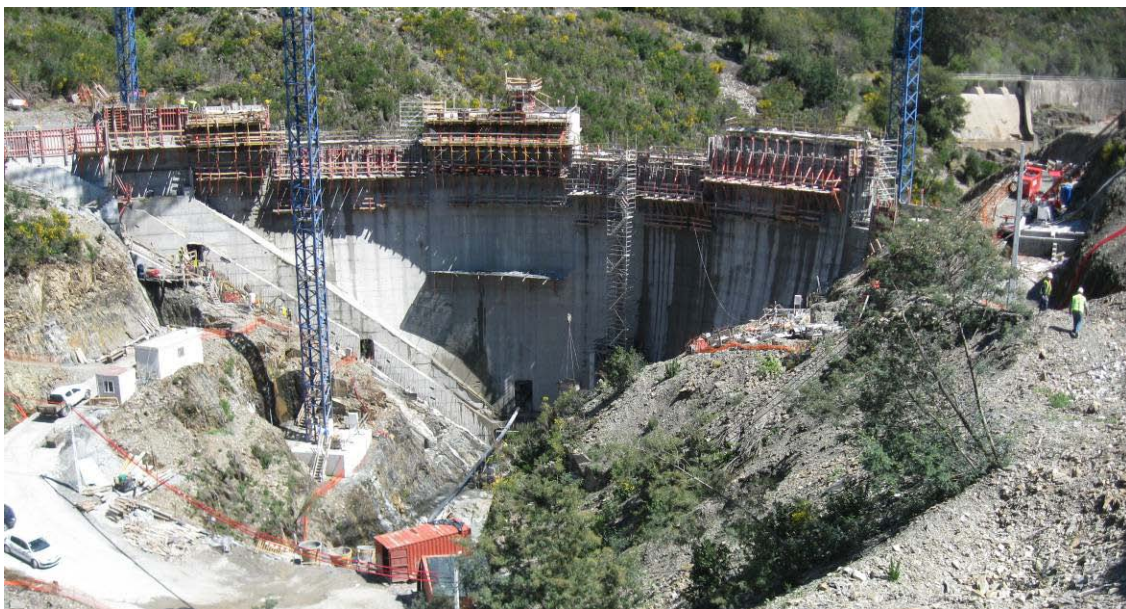
Figure 4 – Downstream view of the New Alto Ceira dam during construction
