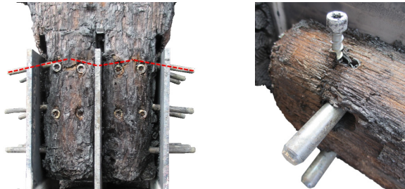
Figure 10: Failure modes of connections D03.1.R-1 (left) and D05.1.R-1 (right) in the fire tests.
