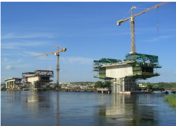
Fig. 2 – Balanced cantilever erection
