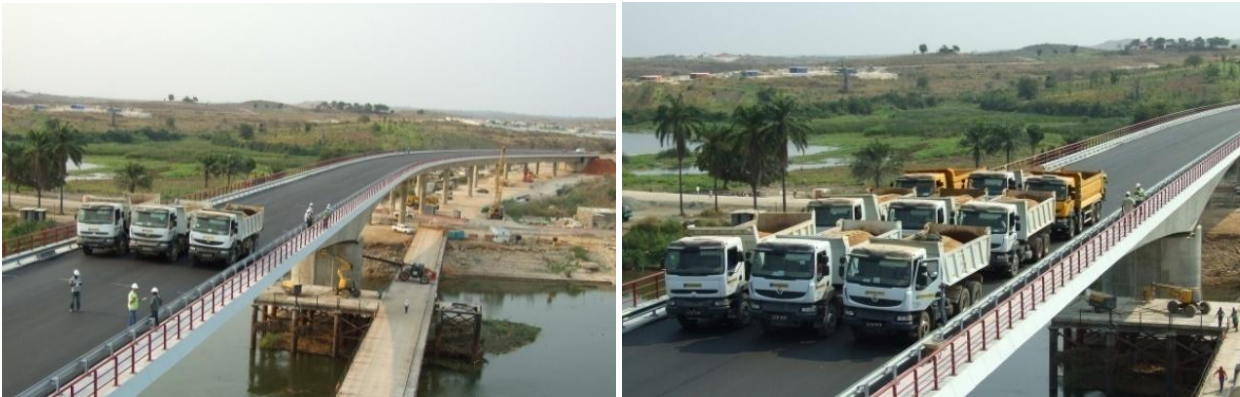
Fig. 13 – Lorries during the static load test
