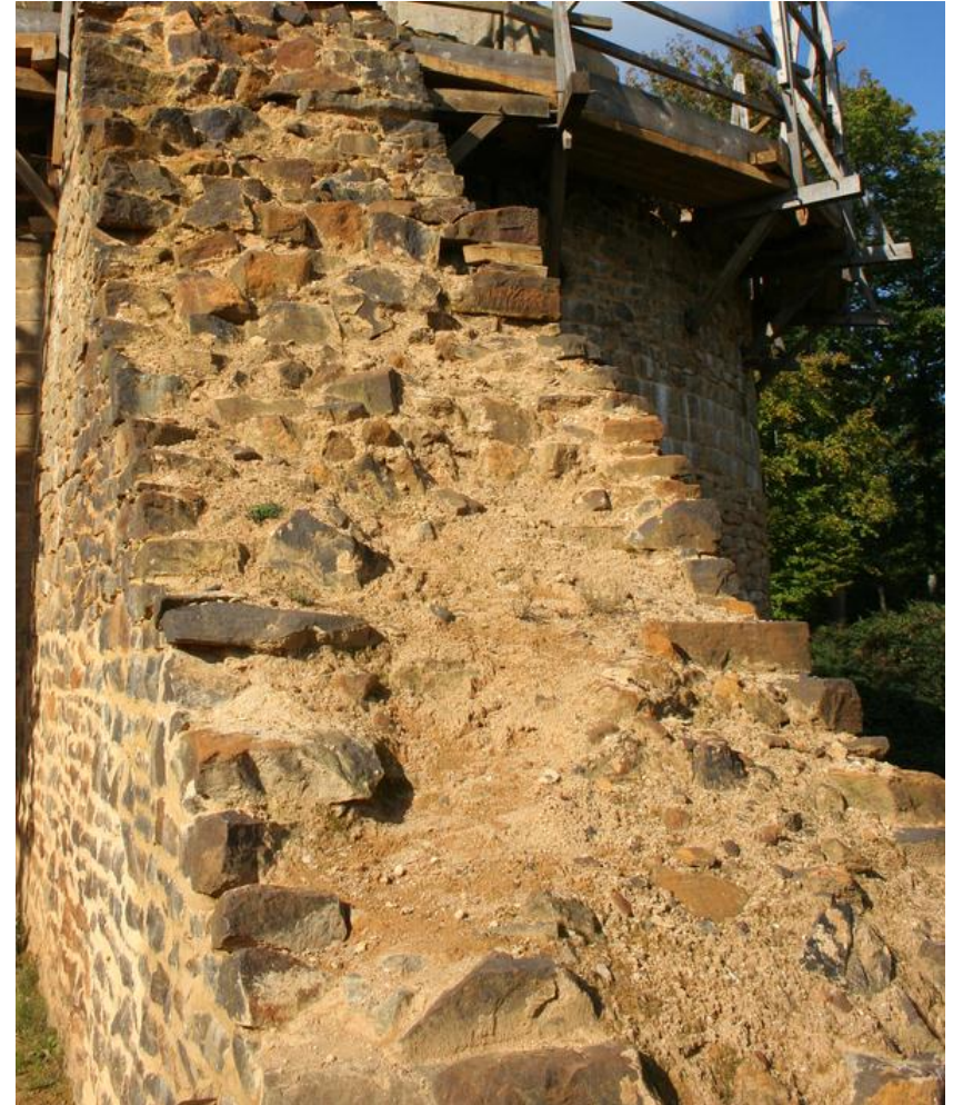
Earth: bedding mortar
