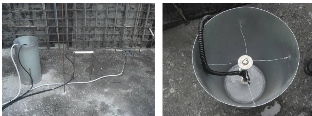
Figure 12 – Double-wall bucket for no stress concrete monitoring (left), and single strain transducer (right).
