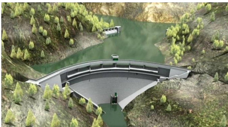
Figure 2 – Preview of the new Alto Ceira dam.
