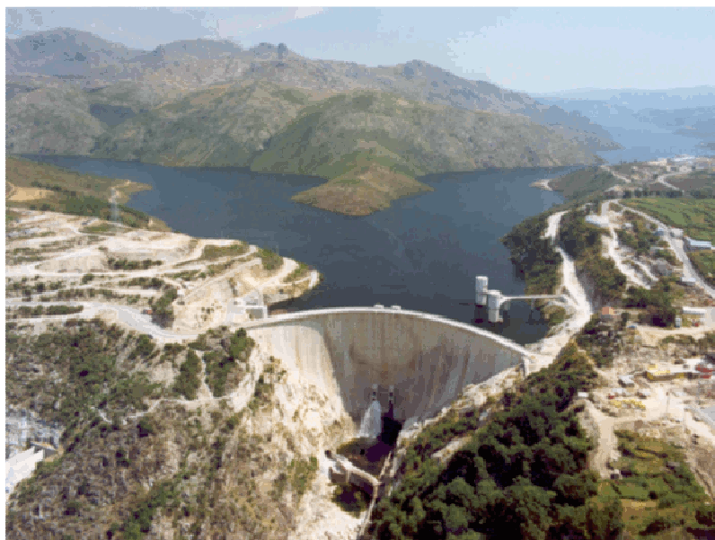
Figure 5 – Alto Lindoso dam.
