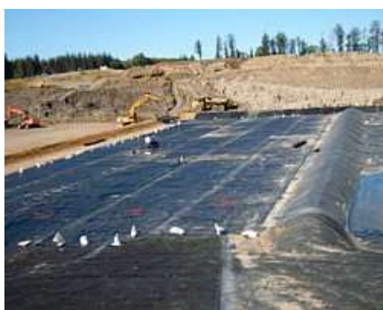
Figure 1: Landfill facility with a barrier system.
