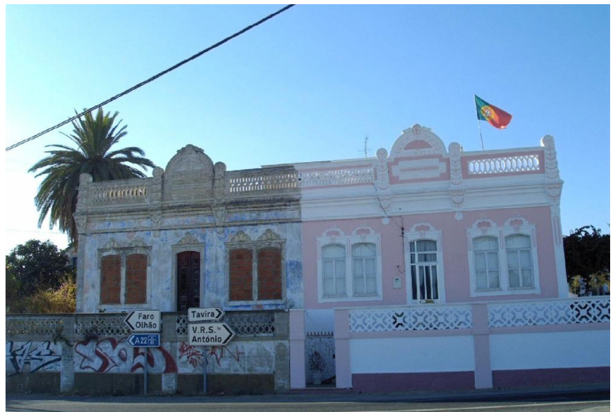
Figure 1 Renderings: before and after restoration
