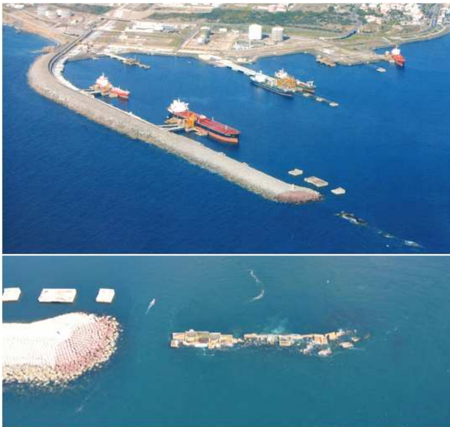
Figure 6: Sines West Breakwater: layout after last rehabilitation works (including remains of the original breakwater)
