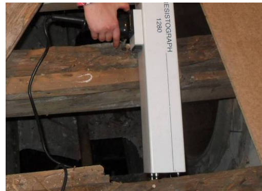
b. Resistograph in Pavement2 beam
