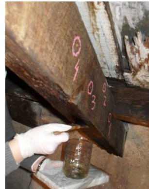
d. Application of consolidant (Roof)
