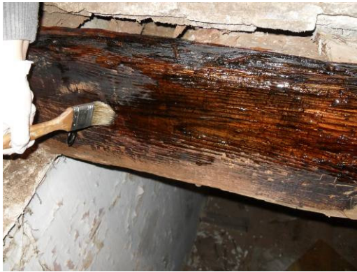
c. Application of consolidant (Pavement2)
