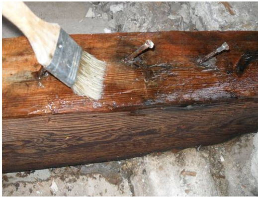
a. Application of treatment product (Pavement1).
