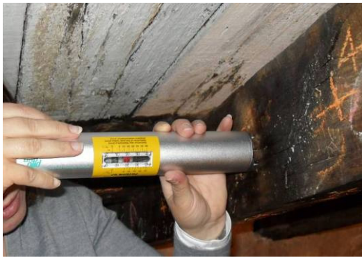
a. Pilodyn test in roof beam
