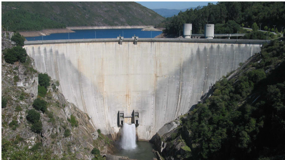
Figure 6: Downstream view of Alto Lindoso dam
