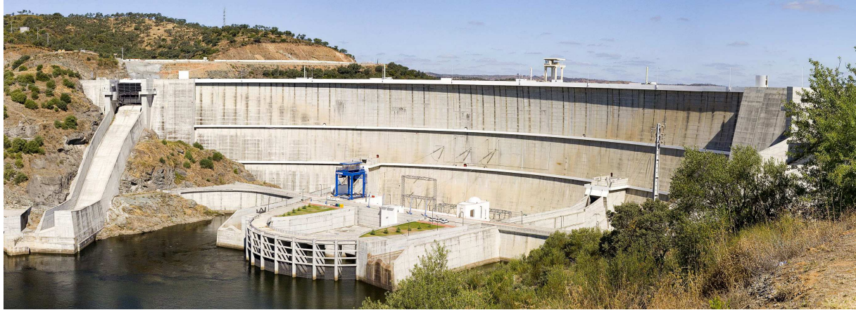
Figure 16: Downstream view of Alqueva dam
