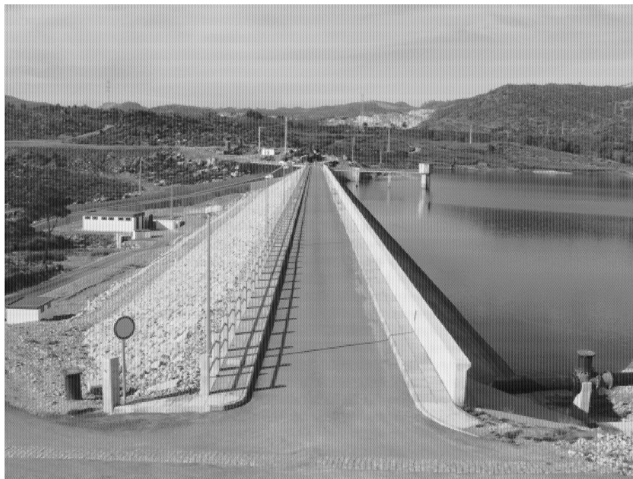
Figure 1: View of Pinhão dam from the left abutment
