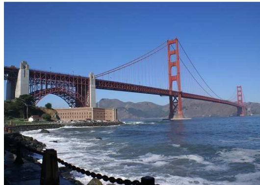
Figura 19 Ponte Golden Gate [1]
