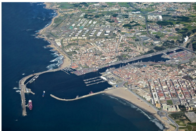
Figure 1. Leixões harbour aerial view (from www.apdl.pt).
