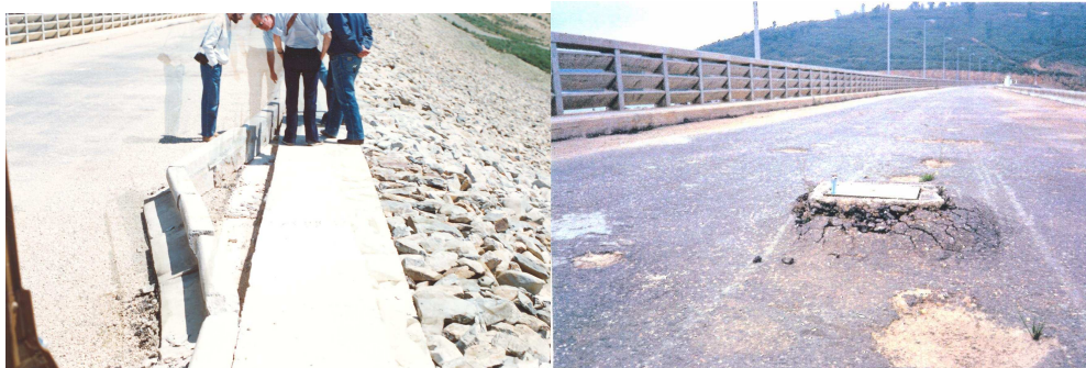
Figure 6 – a) Displacement of the footway beam; b) settlement of the crest pavement
