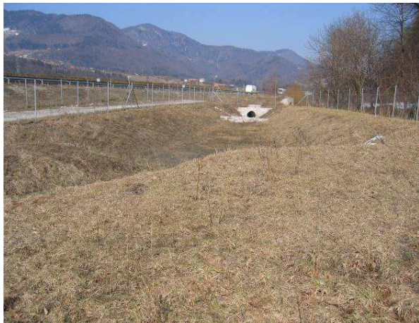
Figure 4 - Ground retention pond along the highway Trojane Vransko – Central Northeast Slovenia
