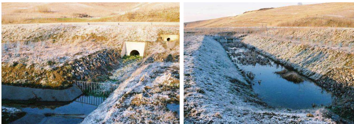
Figure 2 - Example of a detention pond with a system for oil retention, based on a manual process: the closing of a pipe. Highway in Southern France, near Toulouse (Barbosa, 2005); left: Inlet to the system, right: Pond with high L:W ratio
