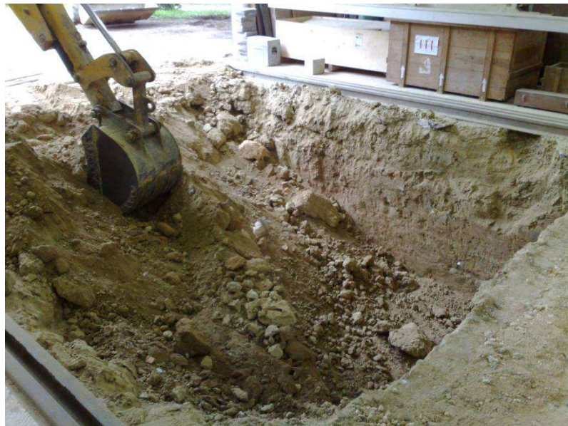
Figure 4 - Excavating works in the rectangular section
