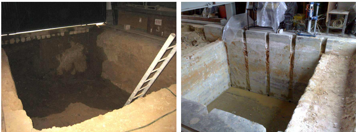
Figure 6 - Fully excavated sections
