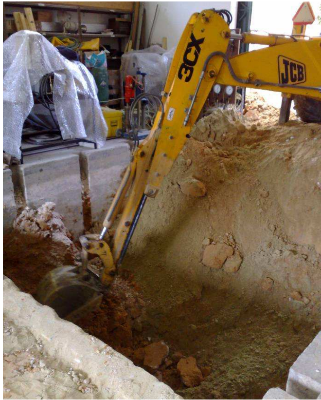
Figure 5 – Excavating works in the concrete pit section
