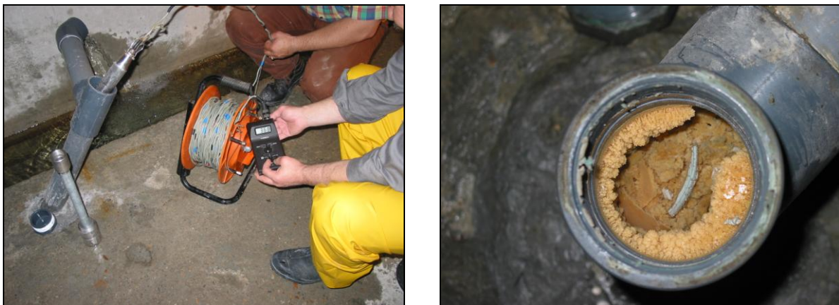
Figure 4.41 – Inserting the conductivity probe inside the borehole and a clogged borehole.
