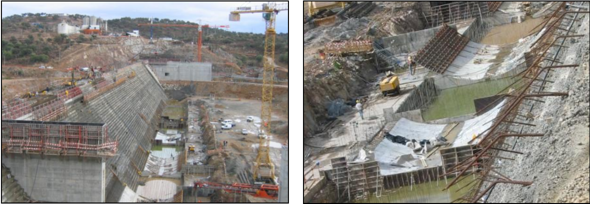
Figure 7.26 – Construction of Pedrógão dam stilling basin.
