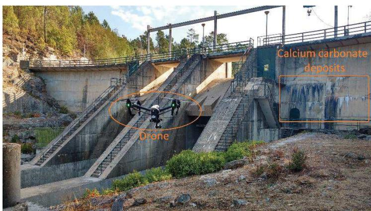
a) UAV (drone) visual inspection of dam with efflorescence ( $\text{CaCO}_3$ )
